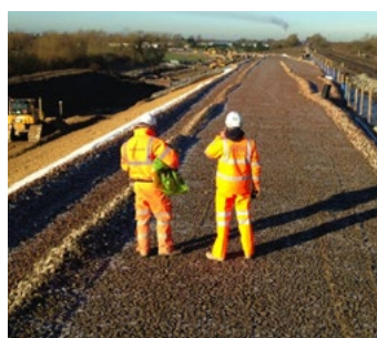
^ Bicester chord bottom ballast and track installed
