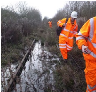
^ Temporary drainage will be installed and the water table level monitored over different seasons.
