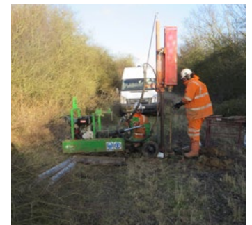
^ Borehole drilling
