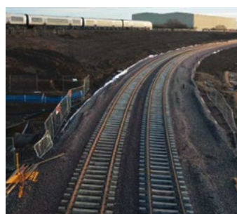
^ Bicester chord bottom ballast and track installed
